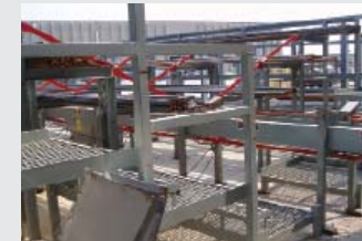
Outside Yard houses stock. Entry table saves operators from lifting bars.
