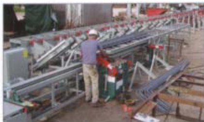
The KRB Rebar Shop
