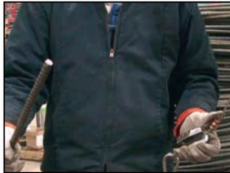
Operator places end of coiled bar into bar guide...
